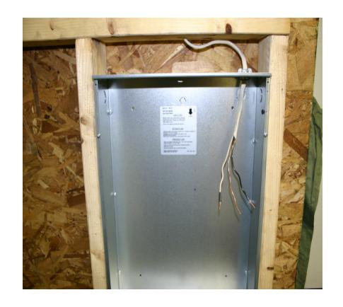
Ground the back box by connecting the supply ground wire to the green ground screw located in the inside top of the back box.
