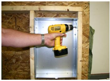
Remove the knockout (KO) in the top of the back box and install a cable clamp.
