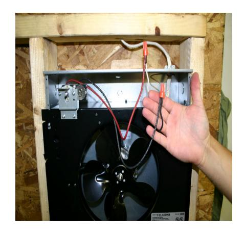
Once all connections have been made and checked, push the wires back into the back box as shown.
