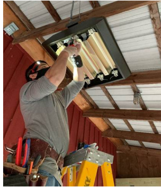
Installation of Marley Infrared Heaters
